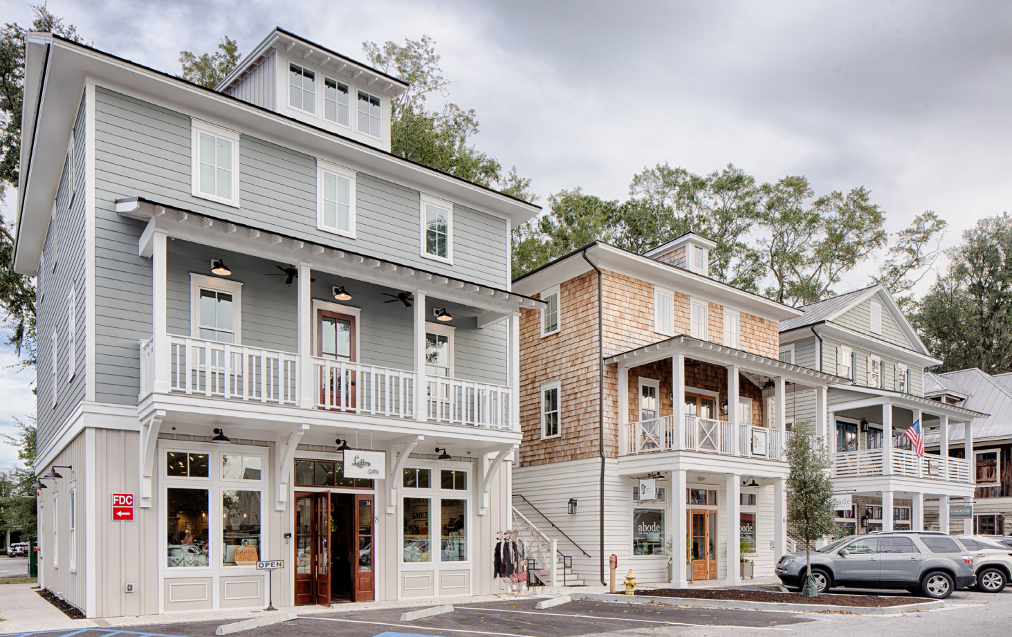
Above, Streetscape of the Promenade in Old Town Bluffton.
