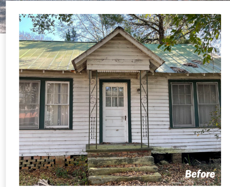
BUILDING ON LEGACY The renovation of the Joiner Homestead artfully preserved its historical essence by reusing many original materials. Salvaged siding, roof panels, brickwork and wrought-iron columns were carefully integrated into the new structure.
