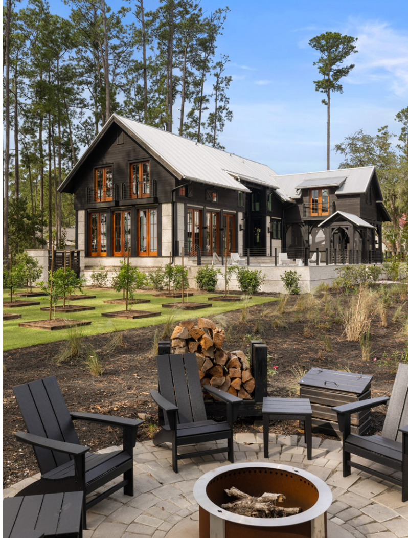
(above) The exterior is tabby stucco in between heavy timber with a corrugated metal roof for a rustic barn-like appearance.
